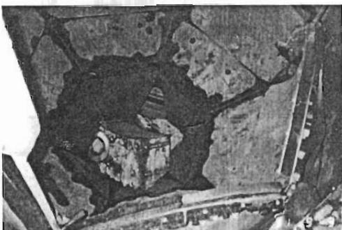
Photo. 3 Recovery of Cutoff Concrete Blocks.
