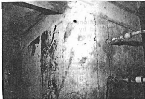
Photo. 7 Crushing by Hydrostatic Tube.
